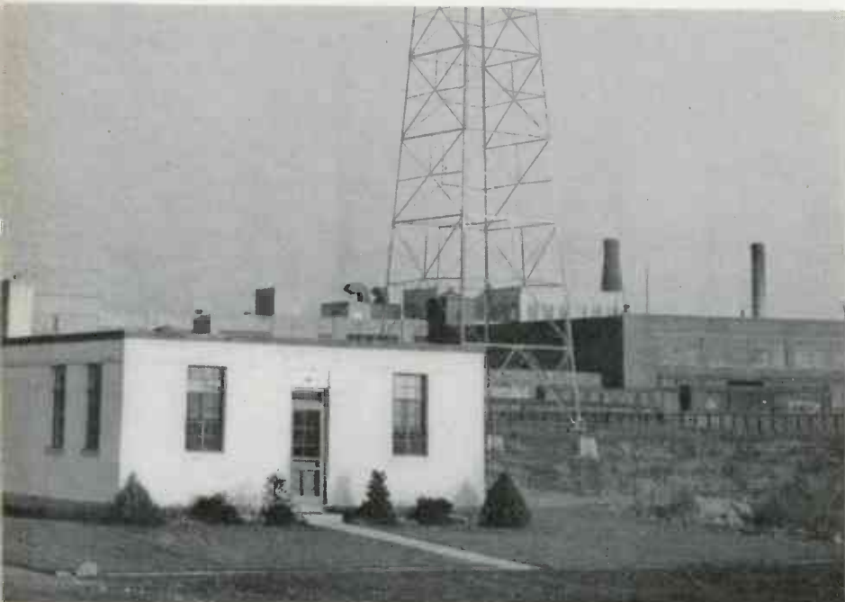
WQXR's transmitter house and tower at Maspeth, L. I.
