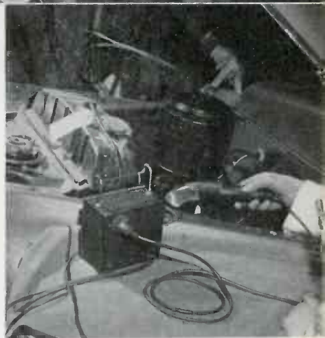
TIMING spark with neon stroboscope
